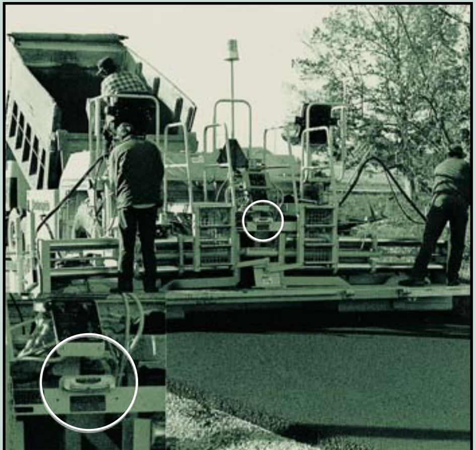
Paving (Photo courtesy of Cedarapids, Inc.)
